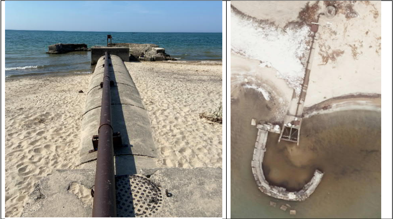
Figure 13 Oil Mill Creek Outlet Structure
