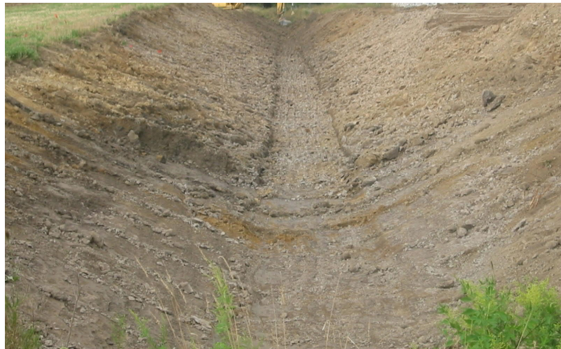
Figure 6 Trapezoidal Ditching Under Construction
