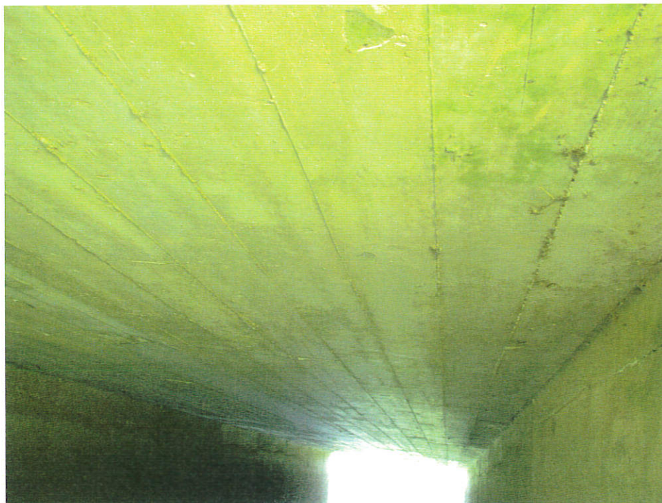
The underside of the structure
