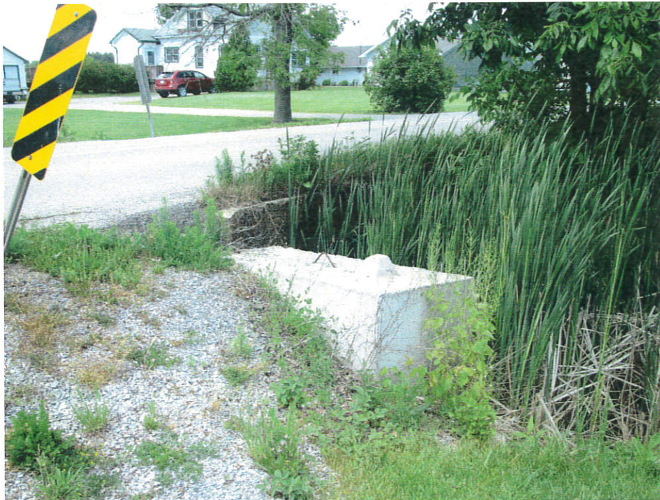
The east end of the structure
