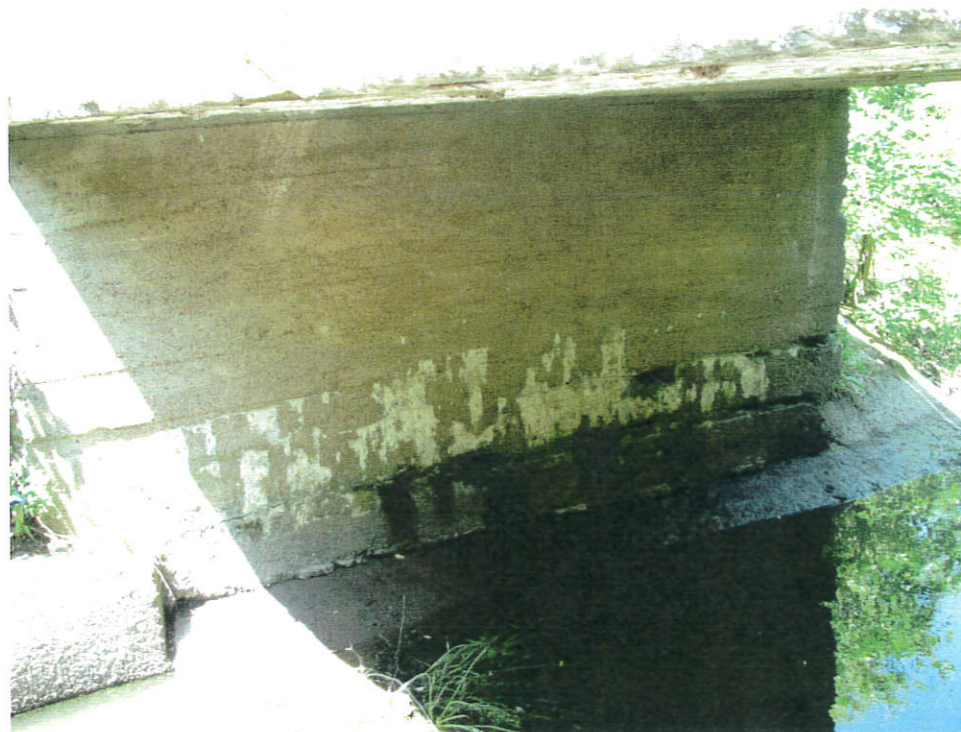
The west wall of the structure
