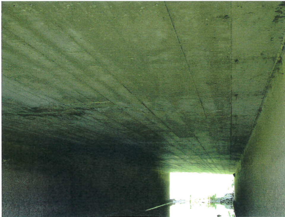
Viewing the interior of the structure, from the south end
