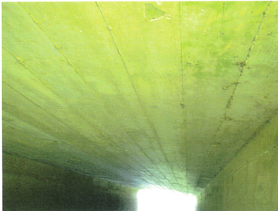
The underside of the structure
