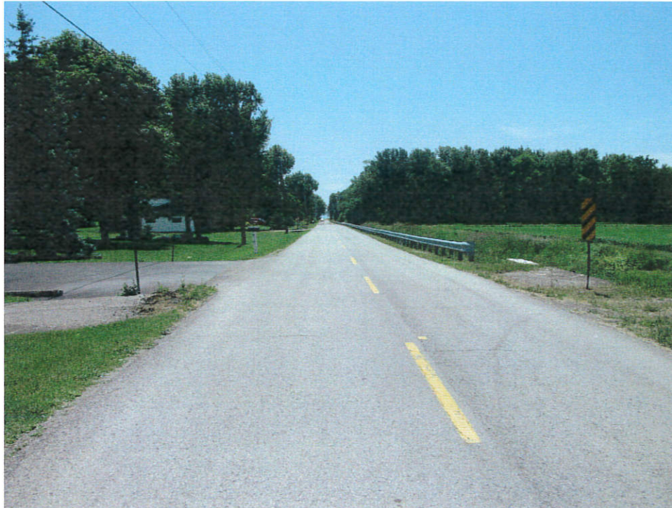
Roadway over the structure - Looking south
