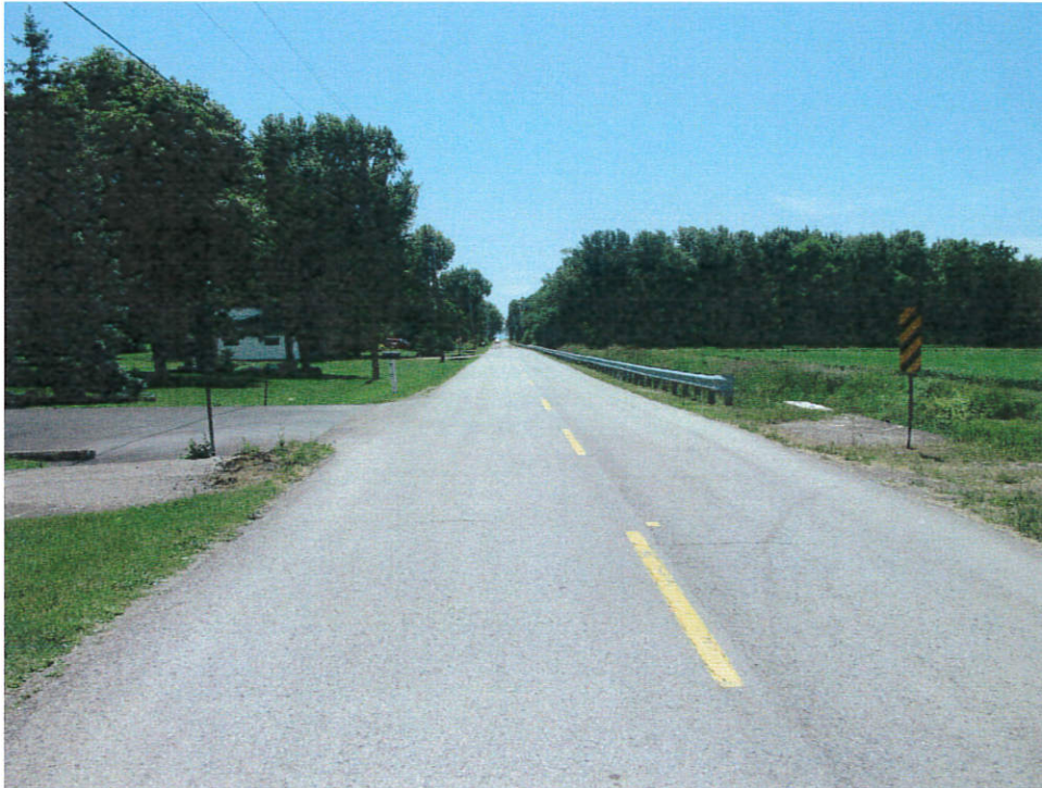
Roadway over the structure - Looking south
