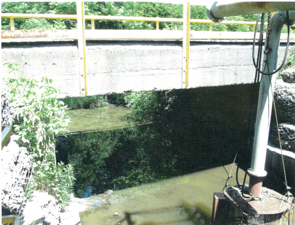
The south side of the structure
