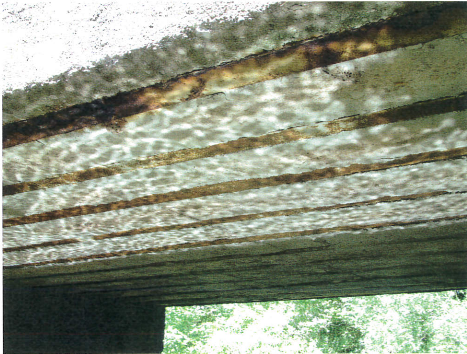
The underside of the structure
