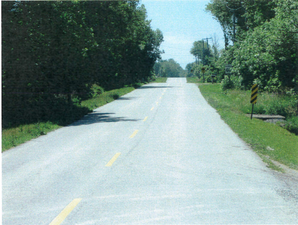
Roadway over the structure - Looking south
