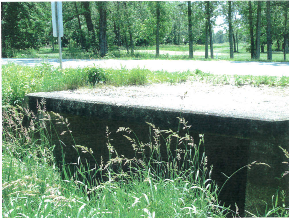
The north end of the structure
