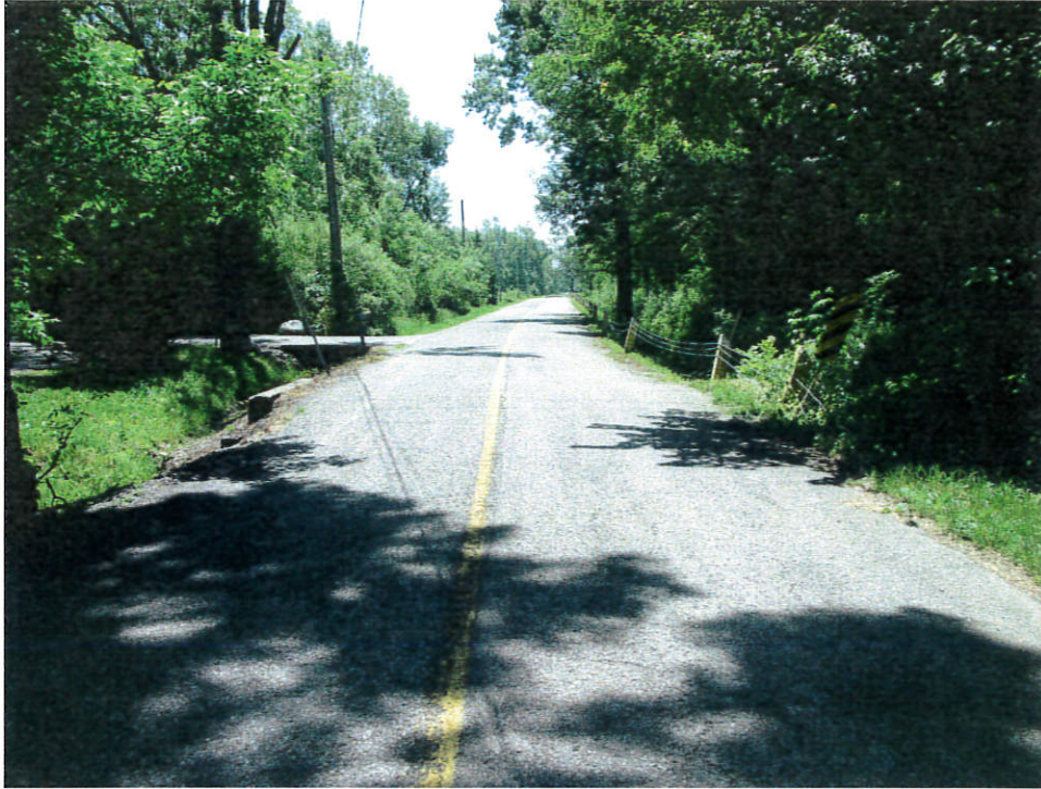
Roadway over the structure - Looking south
