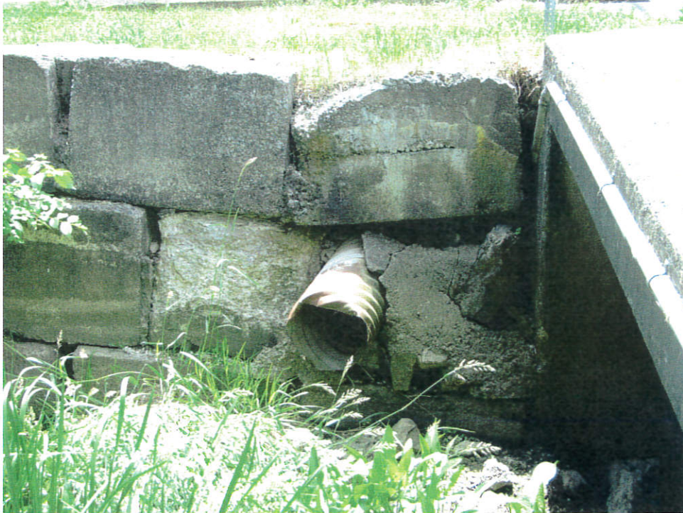
Concrete block retaining wall at the southeast corner of the structure
