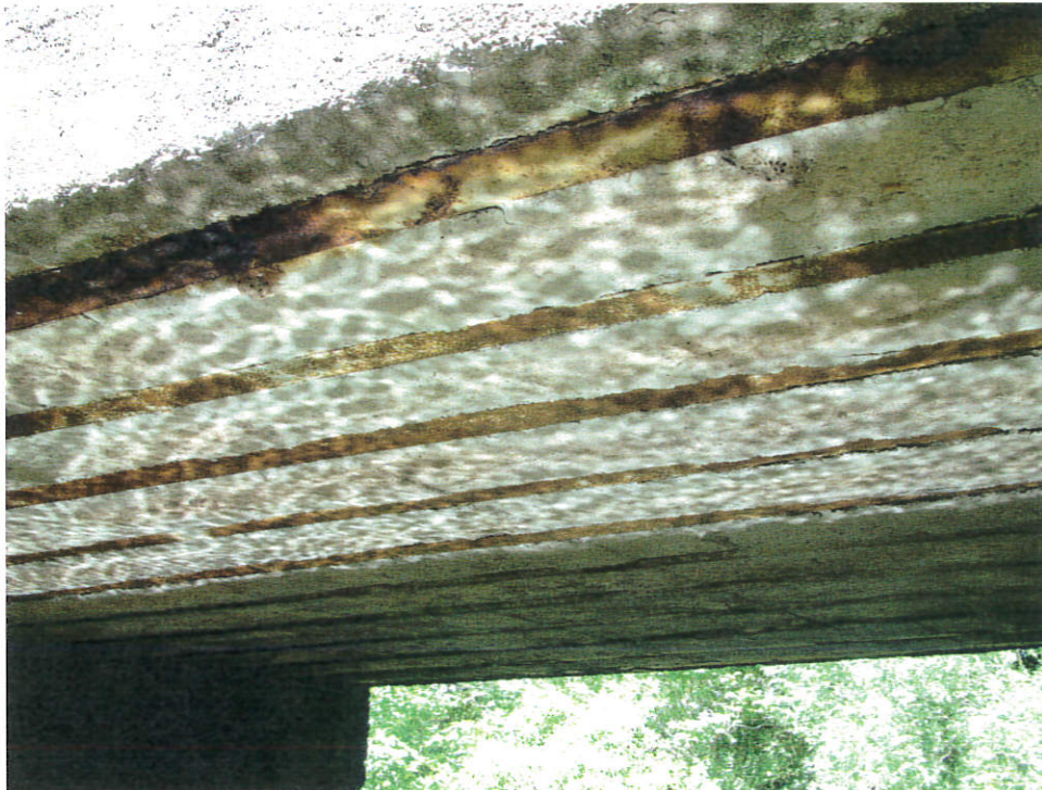
The underside of the structure
