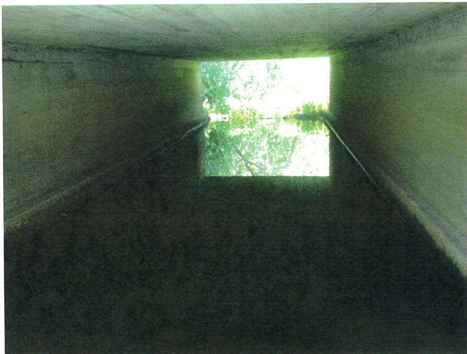
View of the interior of the structure, from the east end
