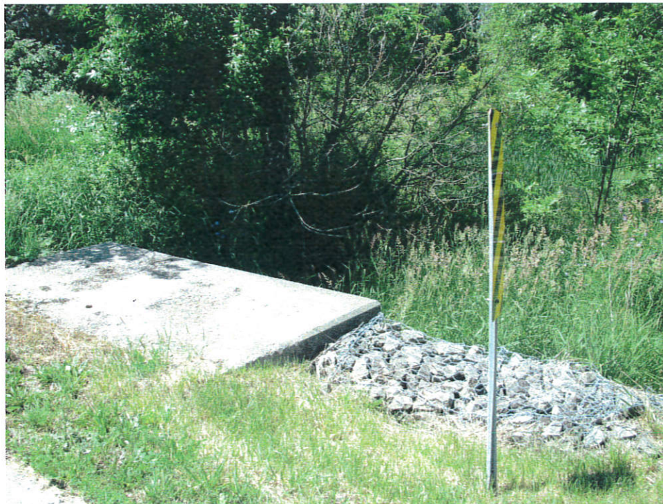
The west end of the structure
