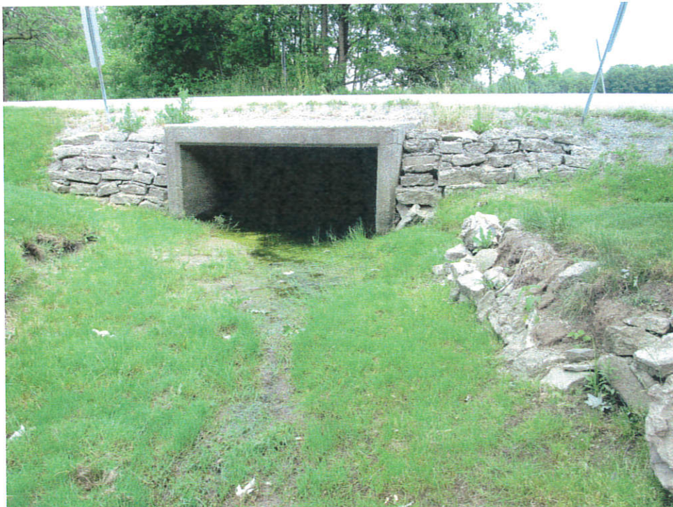
The west end of the structure
