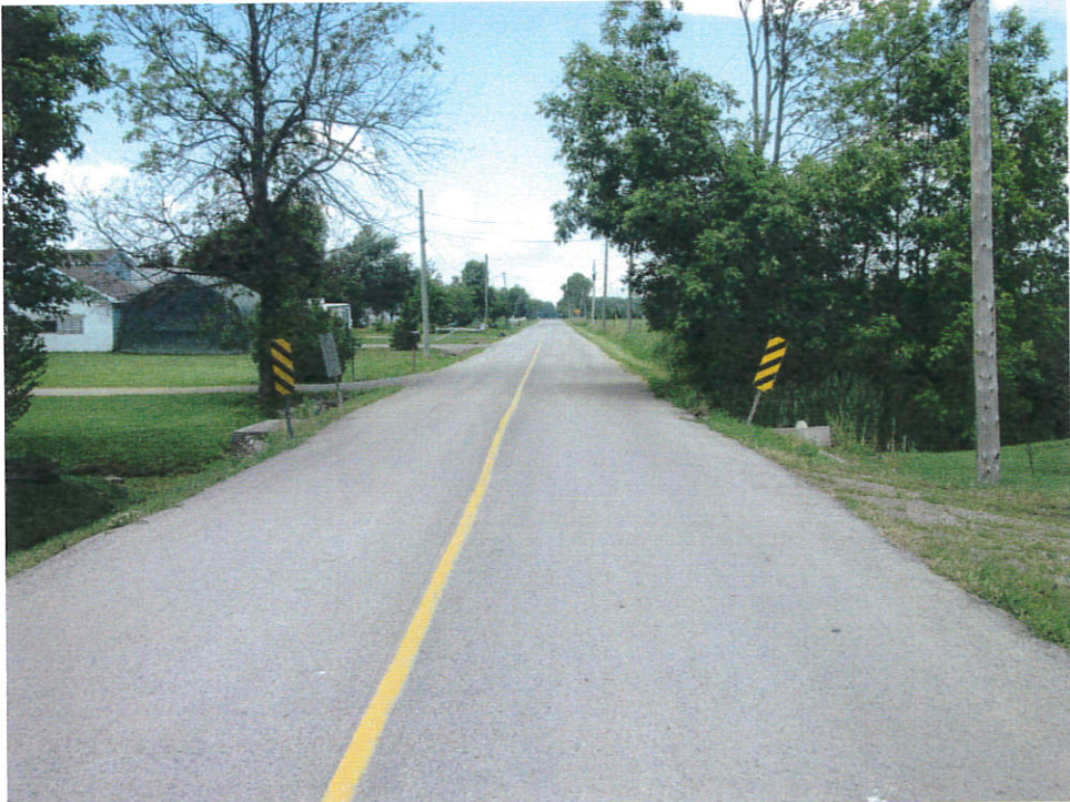
Roadway over the structure - Looking north
