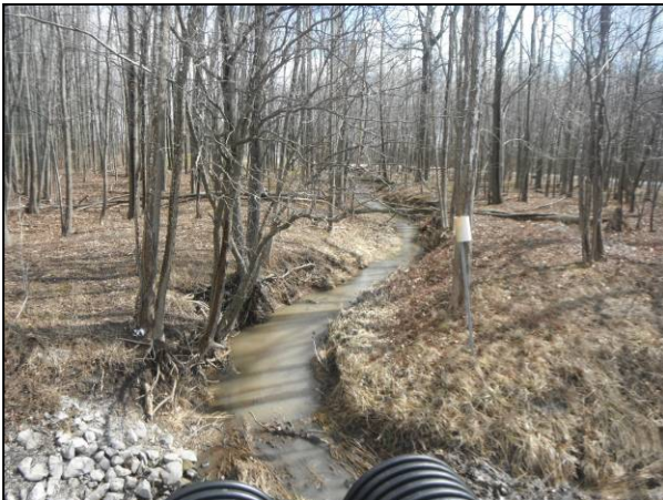
Photo 62: Reach 14-B, channel character, Miller Road cross culvert at point of discharge of roadside ditching system into the West Branch of Beaver Dam Drain.
