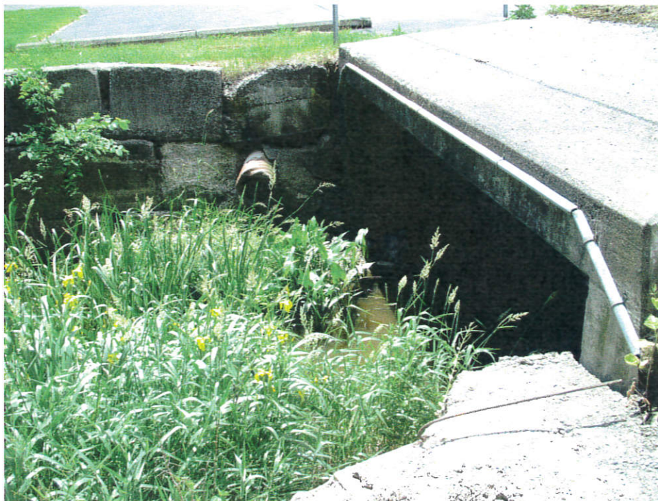
The east end of the structure
