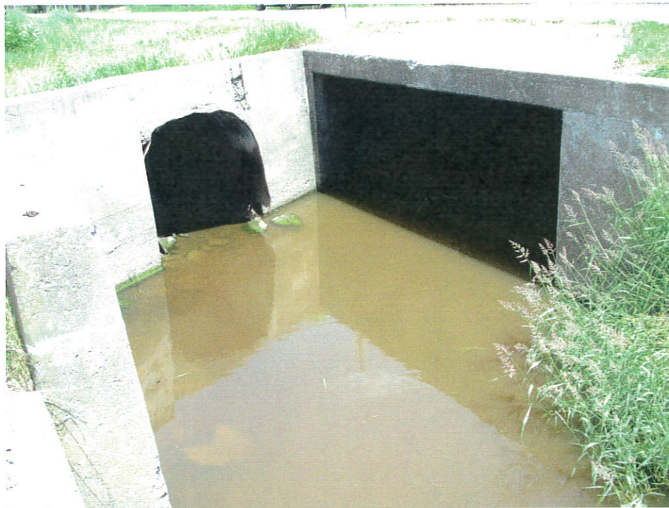
The west end of the structure
