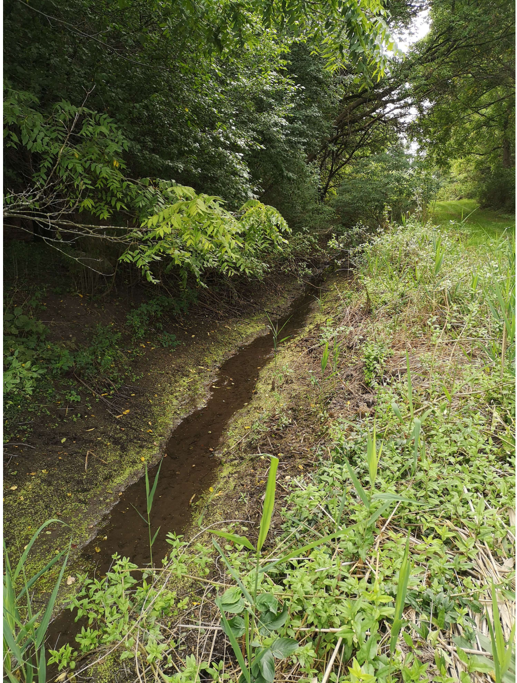
Figure 16 Michener Drain Looking South to Section 2 STA 0+400
