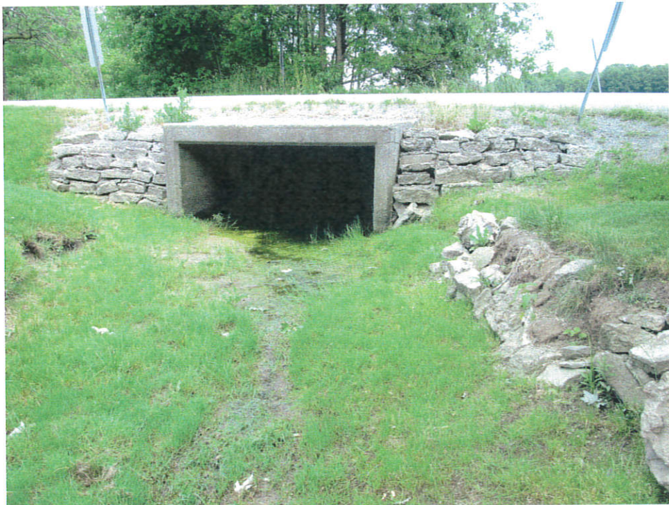
The west end of the structure
