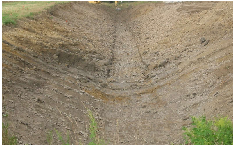
Figure 10 Trapezoidal Ditching Under Construction
