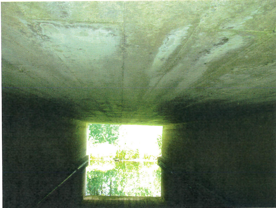
View of the interior of the structure, from the west end
