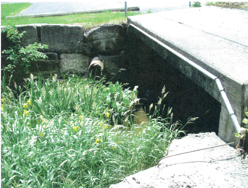
The east end of the structure
